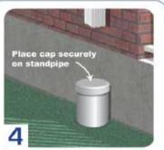
Cap the standpipe where it enters the ground. This prevents any debris, water or small animals from getting into the system and causing a blockage.
