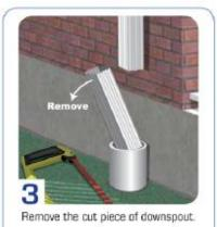
Start by measuring nine inches up the pipe from where the downspout enters the standpipe.
