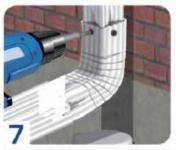
Drill holes and secure the elbows and extensions with sheet metal screws. (self tapping screws have a sharp end so you don't need to pre-drill a hole) One screw on each side is typically enough. (two to four screws)
