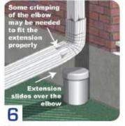
Measure, cut, and attach any needed extensions OVER the elbow to prevent leaking.
