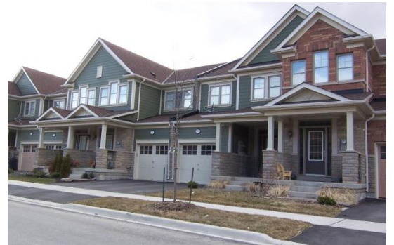
Example of Front Loaded Townhouses with Wall Articulation, Recessed Garages, and Massing Variety
